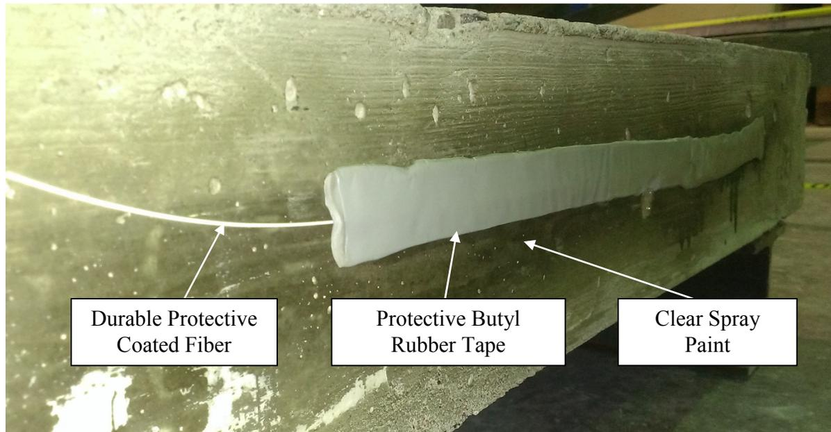
**Figure 3.6 – Protection Method 2 for Fibers Installed on Concrete**
